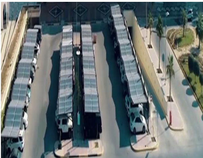
Figure (5) PV Panels Installation for Some Zones A and zone B
